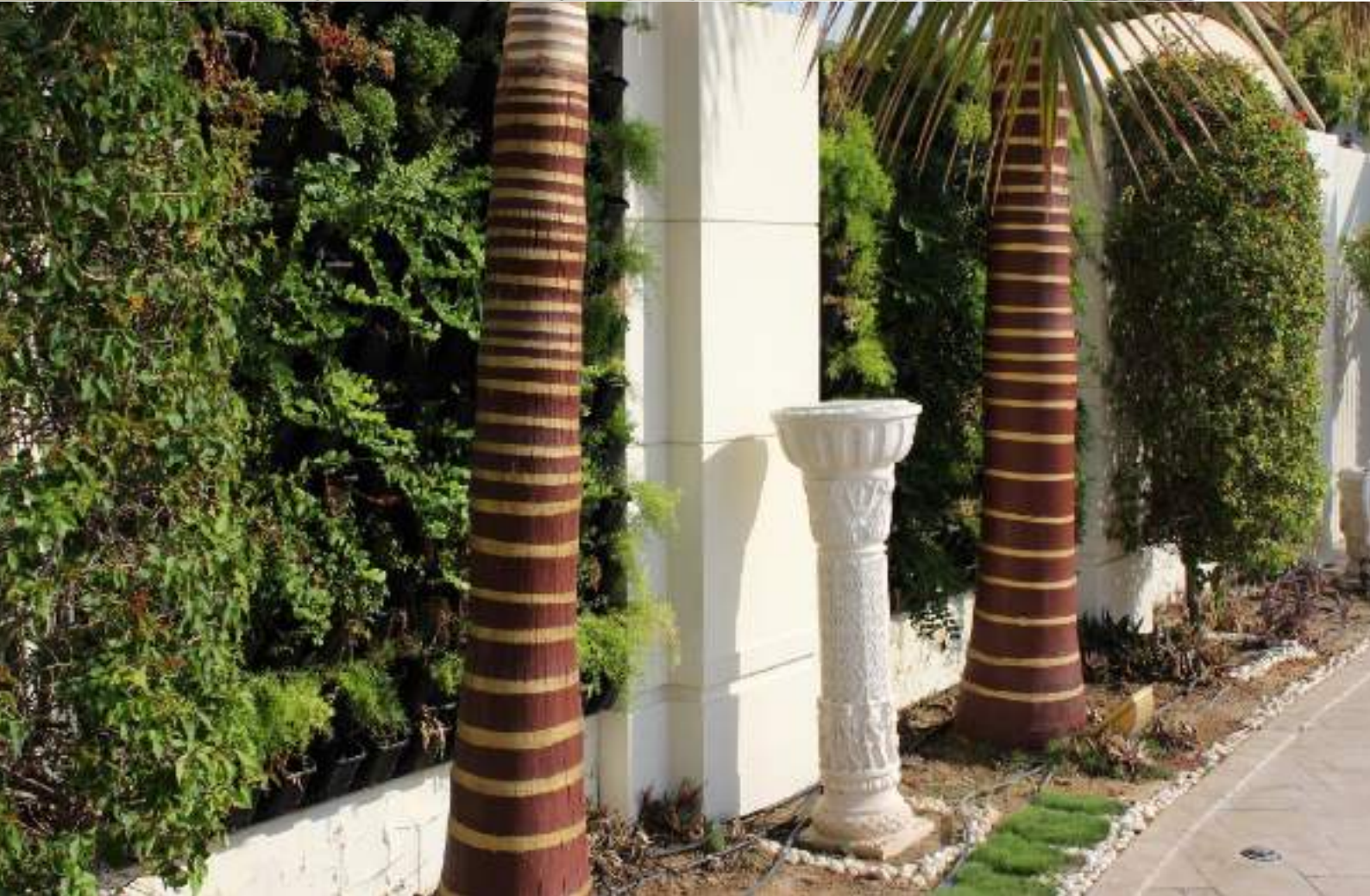
Vertical Garden is a wall partially or completely covered with greenery that includes a growing medium, such as soil. This also features a fully integrated timer controlled drip irrigation system.
